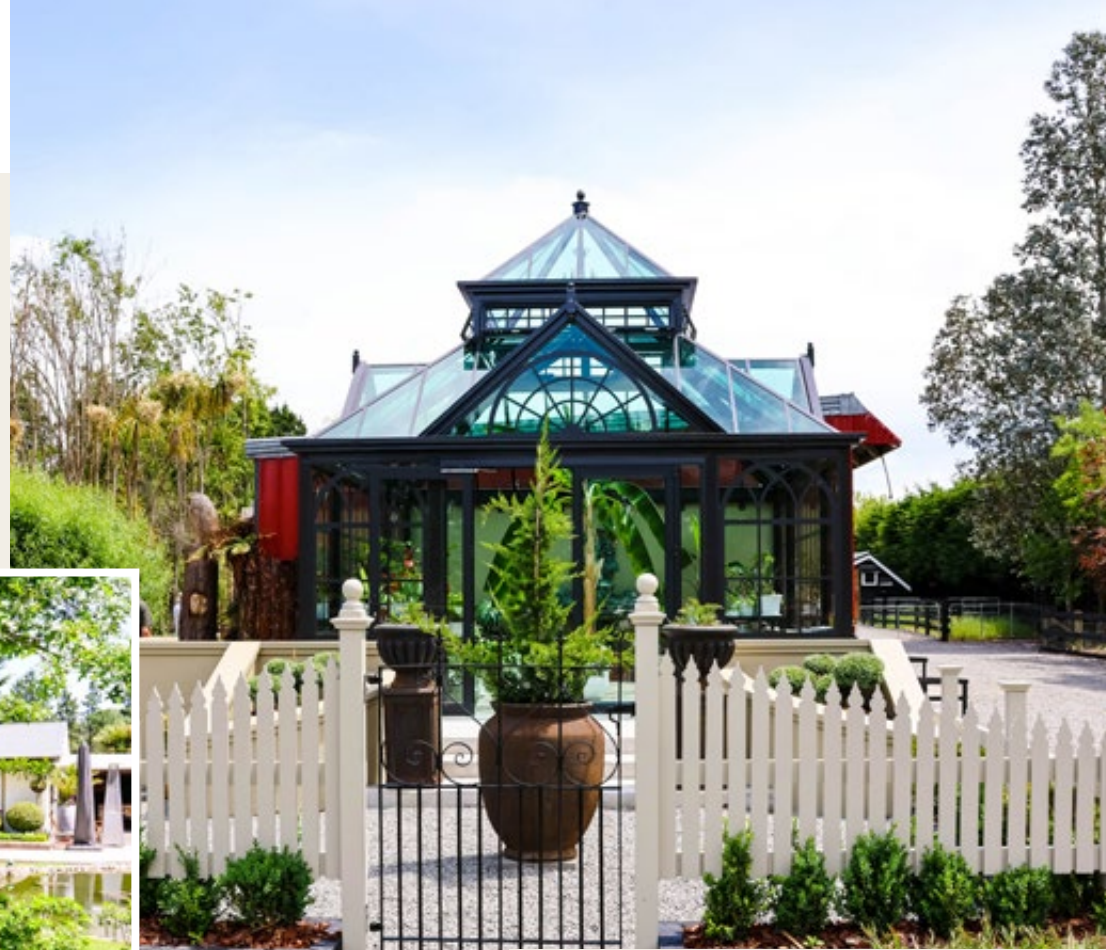
The black steel-framed conservatory has opening air vents at the top to allow heat to escape. It was made by local engineering firm Division Engineering.
