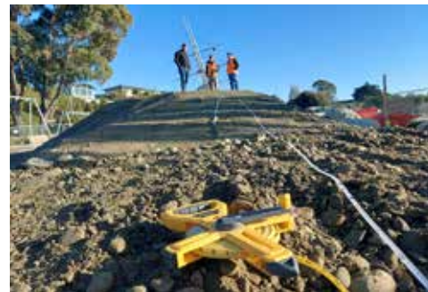
Earthmoving during works. Photo Roselyn Fauth
