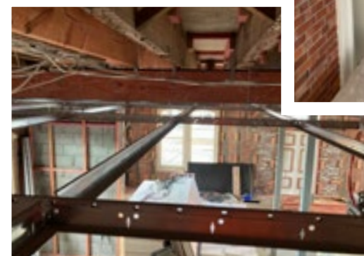
Extensive strengthening work was carried out by Hazeldine Construction including steel framing between the floors.
