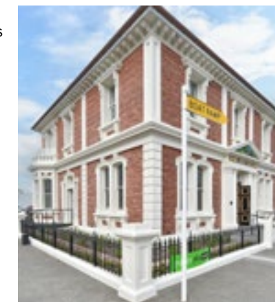
Restoring the BNZ building in Kaiapoi page 18
