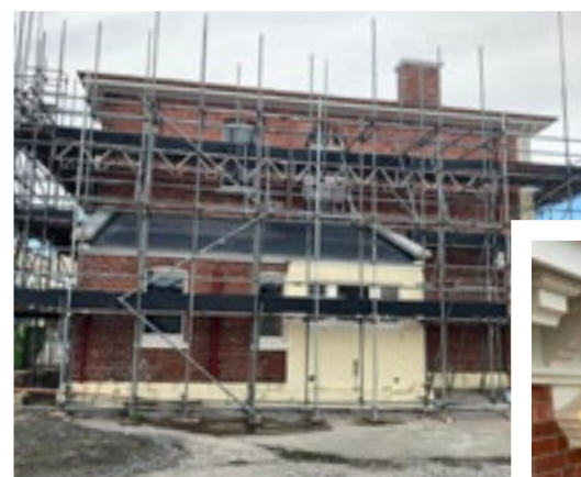
Scaffolding surrounding the two-storey building became a familiar sight in Kaiapoi.
