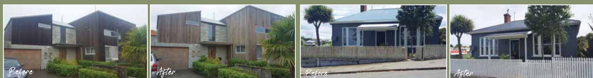
If you have untreated cedar on your home, it can be as easy as a wash down with an oxygen cleaner. It's a natural product easily applied and inexpensive. The before photo is actually a type of mould that is easily removed.
